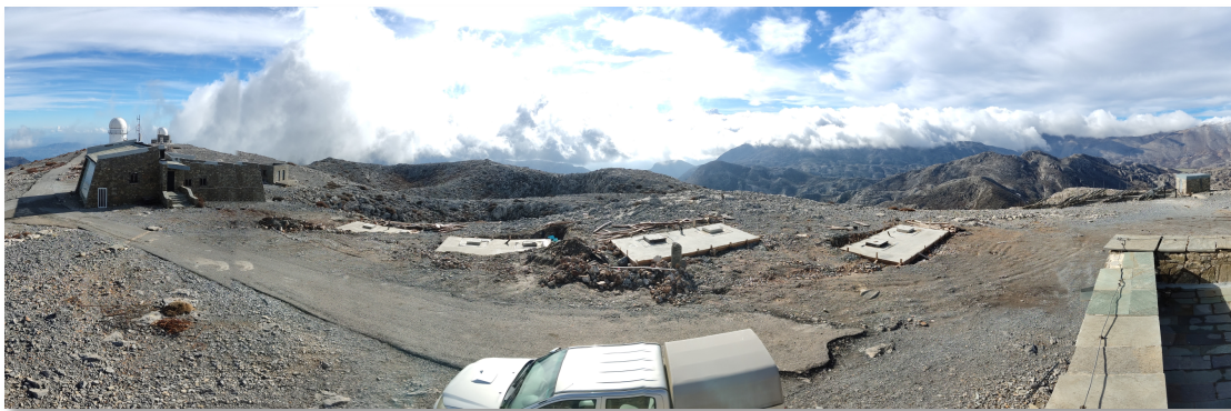
A photo of the four flat concrete bases where the telescope enclosures will be placed (Credit: T. Kougentakis on Dec. 22, 2023).
